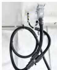
Harting wall bushing M4 inner
