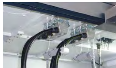
Harting wall bushing K8 inner
